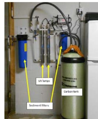
Filtration system installed by Culligan at a home within a mile radius of the CTS site
