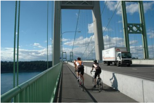
Pedestrian and bicycle path adjacent to the Tacoma Narrows Bridge, Washington
