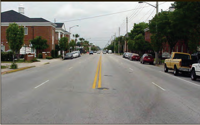
Figure 1. Photo. Four-lane configuration before road diet.
