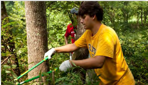
Planned greenway corridors are oftentimes overgrown with weeds, trees and other foliage and need to be cleared not only for trail establishment but to promote safety and visibility along a route.
