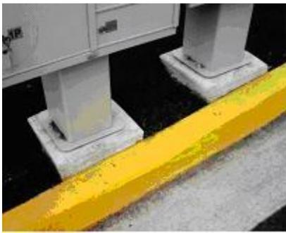
**INCORRECT** - THIS REPRESENTS A SAFETY HAZARD, IS VULNERABLE TO TRAFFIC, AND VIOLATES ADA REQUIREMENTS. THERE SHOULD BE 36 INCHES IN FRONT OF THE CBU FOR WHEELCHAIR ACCESS.
