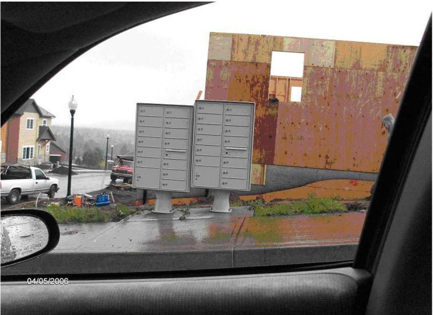
These CBU's are properly installed to be level on this steep hill.
