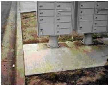
**CORRECT** - TO REDUCE MAINTENANCE COSTS, INSTALL CBU AWAY FROM THE STREET. CBU'S ARE EASILY DAMAGED WHEN INSTALLED NEXT TO THE STREET.
