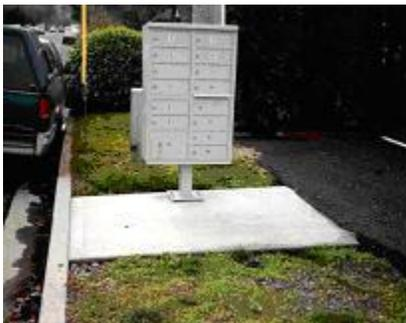
**CORRECT** - IF THIS CBU WAS INSTALLED NEXT TO THE CURB IT WOULD OFTEN BE BLOCKED BY PARKED CARS AND THE CARRIER WOULD NOT BE ABLE TO OPEN IT.
