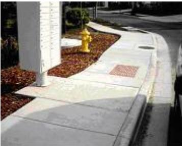
**CORRECT** – PLAN AHEAD. THIS PAD WAS ACTUALLY POURED BEFORE THE SIDEWALK WAS PUT IN. THE DIMENSIONS, ELEVATION, AND SLOPE WERE CALCULATED TO MATCH THE FUTURE SIDEWALK.
