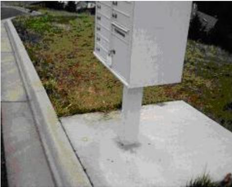
**INCORRECT** - THE PEDESTAL IS EMBEDDED IN THE CONCRETE MAKING THE CBU VERY DIFFICULT TO MAINTAIN.
