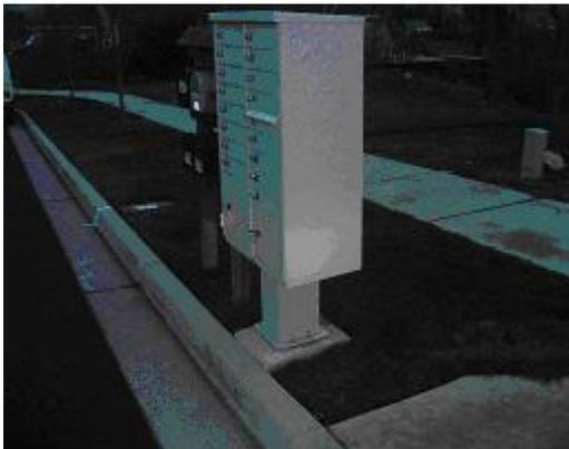
**INCORRECT** - THE CONCRETE PAD ANCHORING THIS CBU IS TOO SMALL. ALSO, THE CBU IS FACING THE STREET. CUSTOMERS SHOULD NOT HAVE TO STEP OFF THE CURB INTO THE STREET TO GET THEIR MAIL.
