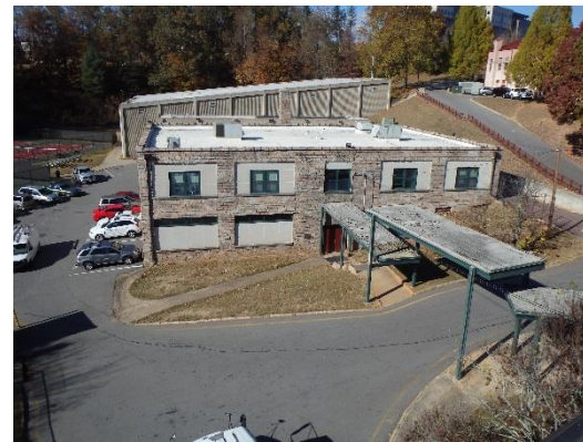
Site Before & After
