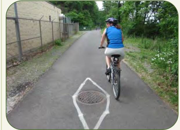
Sewer caps on paved greenways may be flush with the trail but can pose a hazard to bicyclists when wet.
