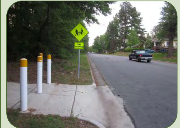
Micropath connections from neighborhood streets to greenways include signage, smooth transition areas and bollards to prevent vehicle use.
