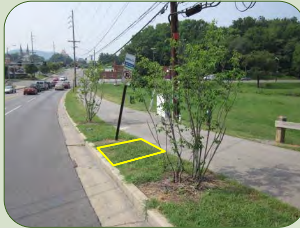
Transit stops along greenways require a paved landing area—minimum dimension of 4' x 4', flat—connecting the pathway to the street. It should have been placed in the area outlined in this image.
