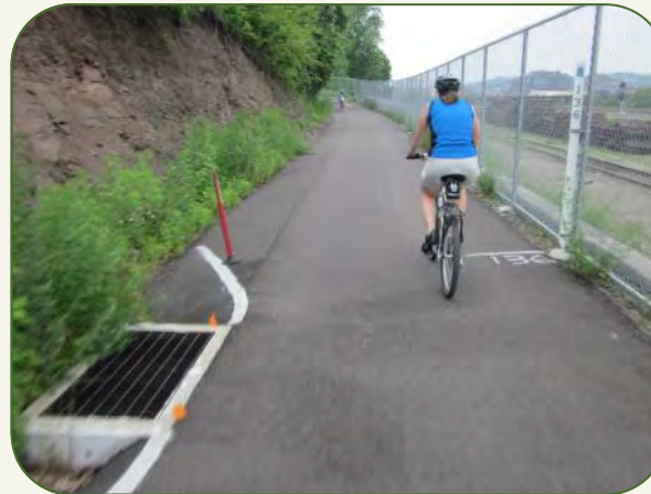
Drainage grates may be necessary to control stormwater and can encroach on the trail. A marking around the grate alerts users to avoid it.
