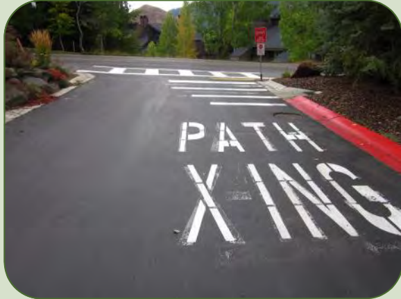
Pavement markings from private driveways alert motorists to expect users to cross in front of them along a sidepath.
