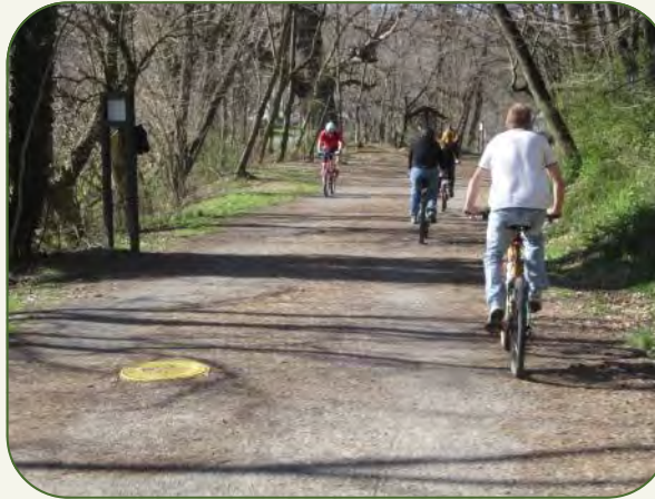
Sewer caps on the Virginia Creeper Trail are not flush with the trail surface. They are painted yellow as a warning for approaching users.
