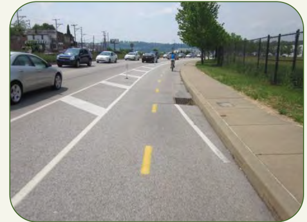
Drainage grates may also be marked with a diagonal line in the direction of travel for trail users so they can avoid it.
