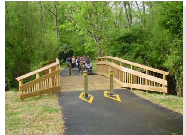
This bridge along the Flat Creek Greenway in Black Mountain represents one of the most common structures along greenway.
