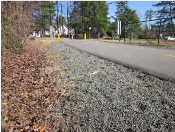
Greenways have to be designed and not simply built. The mounding of a greenway (above), even by just a few inches, maximizes the investment in the greenway by allowing for a better flow of water under the surface, minimizing encroachment of foliage, and protecting the trail surface from root heaves.
