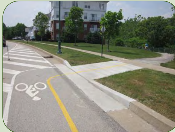
On-street pathways can be used to fill gaps in greenways. The width and radius of the transition needs to consider the speed of bicycles.
