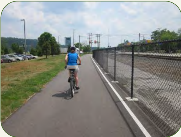
Fences constructed to keep users out of private property can be marked with a line to delineate the clear zone, keeping users away from obstructions along the trail's edge.
