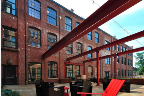
Miller's Court – Baltimore, MD Mixed Use Property Containing Educator Housing and Non-Profit Office Space
