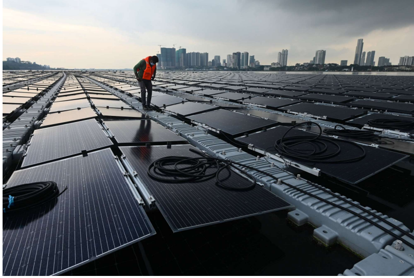
The new frontier in deployment of utility scale solar in urban areas and mountain regions – floating solar (FPV). Photo: Singapore.
