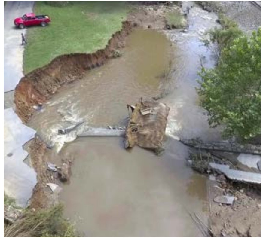
Damage to a road and bridge in Candler following a flooding event.
