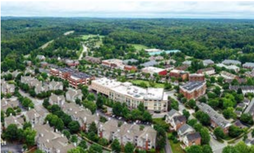
Southern Village in Chapel Hill, NC is an example of a Walkable Destination Center.
