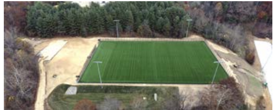
Soccer fields under construction at the Buncombe County Sports Park.
