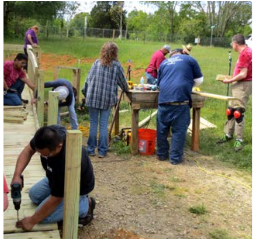
Construction of an ADA ramp through a local repair program.
