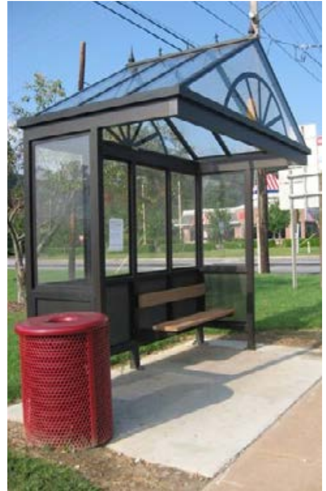
A bus shelter installed in Buncombe County.
