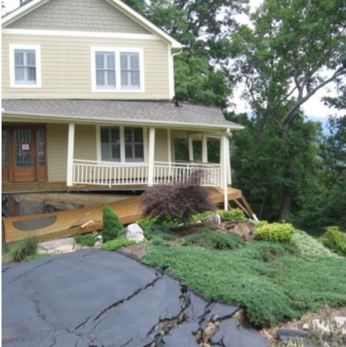
Left: House in Buncombe County with debris from a landslide after an embankment failure, July 2013. Right: Landslide on the Blue Ridge Parkway, 2004. Image courtesy of NC Geological Survey
