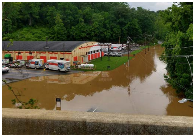
Above: Flood event in May 2018 near the Swannanoa River Road and Tunnel Road intersection in Asheville. Image courtesy of Fernleaf.
