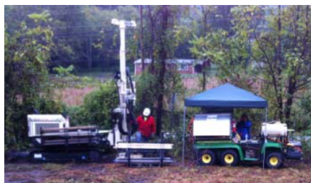
Boring at MHP-02
