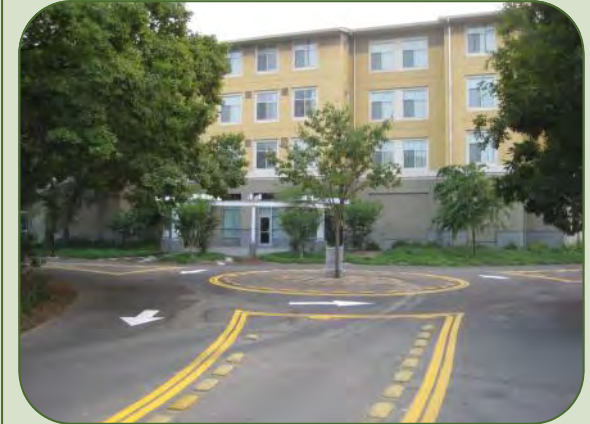
High volume intersections of two pathways may require special design features, such as this greenway roundabout in Davis, CA.
