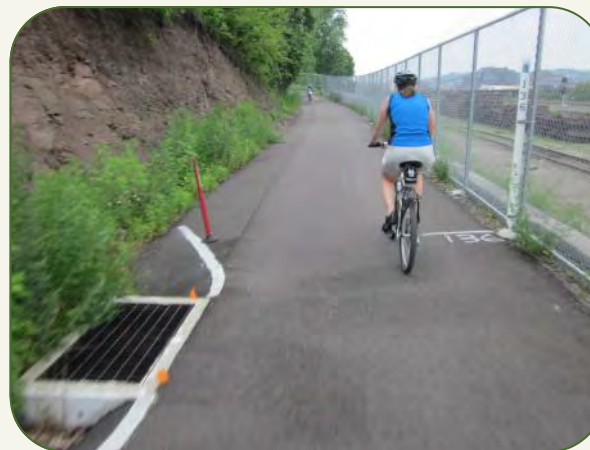
Drainage grates may be necessary to control stormwater and can encroach on the trail. A marking around the grate alerts users to avoid it.
