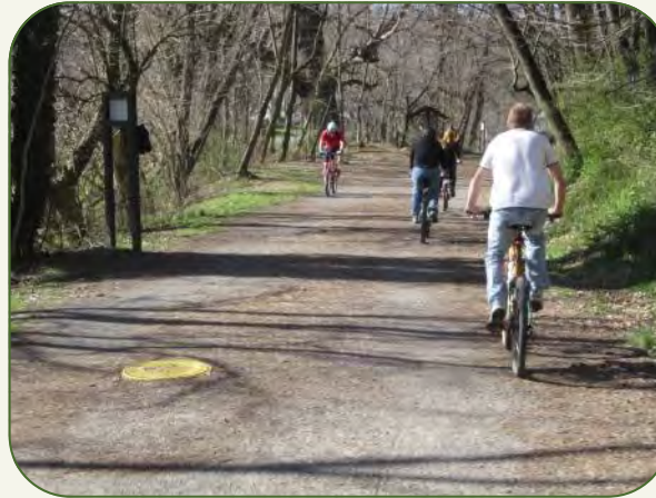
Sewer caps on the Virginia Creeper Trail are not flush with the trail surface. They are painted yellow as a warning for approaching users.
