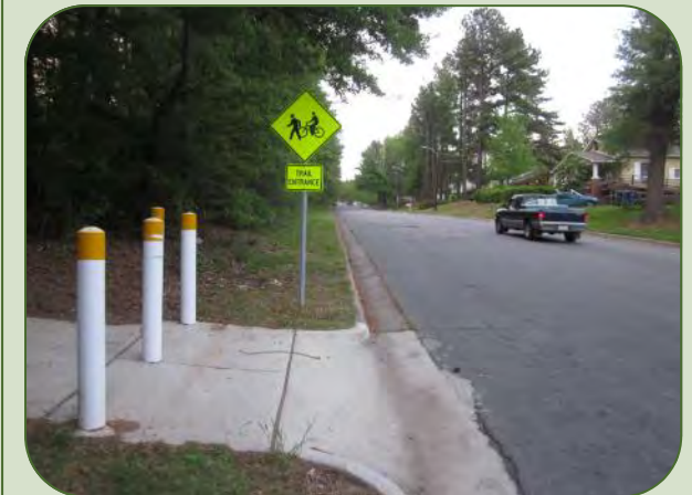
Micropath connections from neighborhood streets to greenways include signage, smooth transition areas and bollards to prevent vehicle use.
