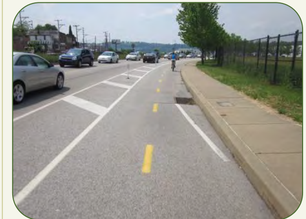
Drainage grates may also be marked with a diagonal line in the direction of travel for trail users so they can avoid it.
