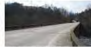
Entrance of Fletcher Street Road to Woodson Park (Looking North)
