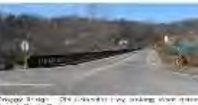
Griggs Bridge - Old Levisa Hwy (Looking East from the Griggs Bridge)
