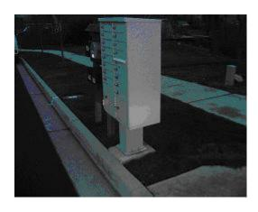
**INCORRECT -** THE CONCRETE PAD ANCHORING THIS CBU IS TOO SMALL. ALSO, THE CBU IS FACING THE STREET. CUSTOMERS SHOULD NOT HAVE TO STEP OFF THE CURB INTO THE STREET TO GET THEIR MAIL.
