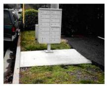
**CORRECT - I**F THIS CBU WAS INSTALLED NEXT TO THE CURB IT WOULD OFTEN BE BLOCKED BY PARKED CARS AND THE CARRIER WOULD NOT BE ABLE TO OPEN IT.
