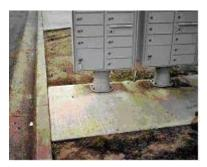
**CORRECT –** TO REDUCE MAINTENANCE COSTS, INSTALL CBU AWAY FROM THE STREET. CBU'S ARE EASILY DAMAGED WHEN INSTALLED NEXT TO THE STREET.
