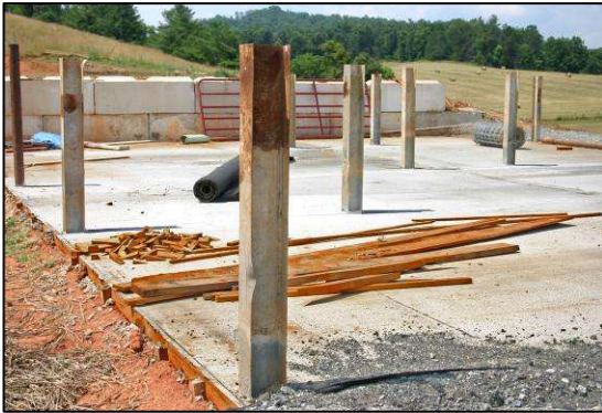
Animal waste storage facility during construction phase in Leicester (cost shared by NCACSP)
