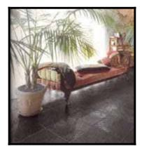
Flagstone: Cut or randomly broken stone that is set in grout or concrete.
