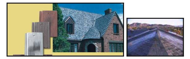
**Tile:** Tile shingles are made of clay that is baked to a hard surface and need no paint. The tiles usually are a half circle shape and are the color of clay (red, brown, or rust).
