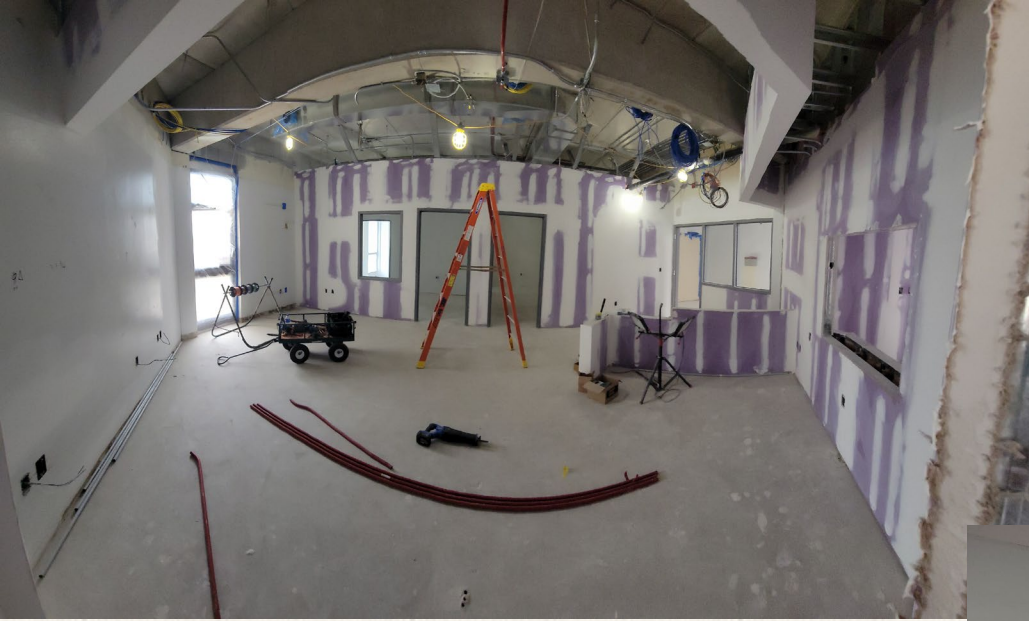
UNDER CONSTRUCTION JUNE 2022
