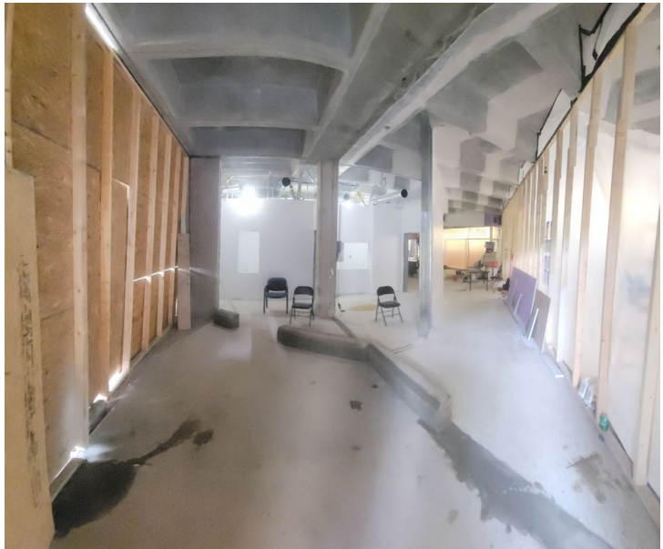
UNDER CONSTRUCTION JUNE 2022
