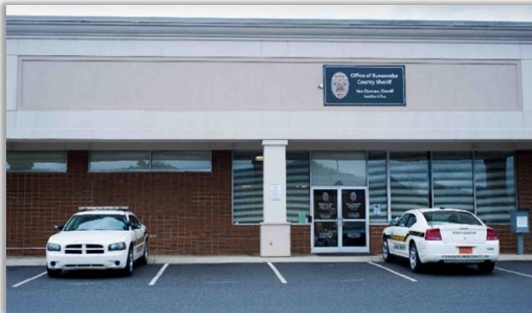
Sheriff Evidence Room New Location - Leicester Highway
