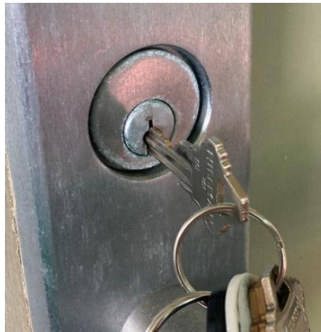
Key hole changed shape in ELC door, no longer fits.
