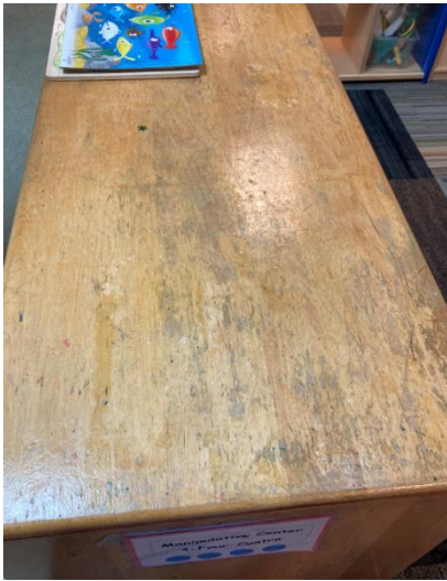
Top of table varnish came off in ELC classroom.
