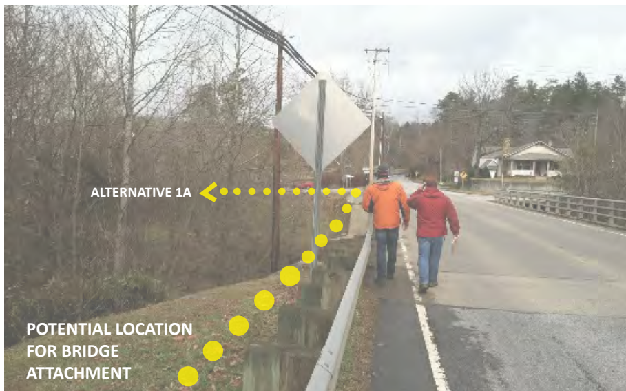
The bridge crossing of Merrimon Avenue over Reems Creek currently does not accommodate pedestrians and bicyclists.
