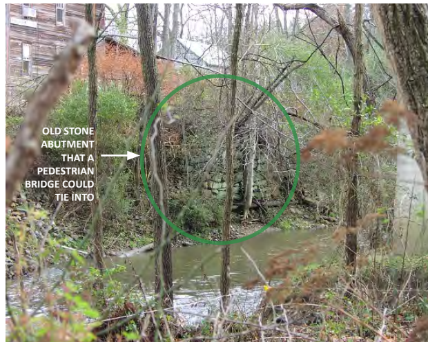
A view across Reems Creek to the Mill and a "historic" abutment made from stone.
