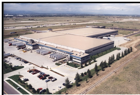
Cold Storage Warehouse
