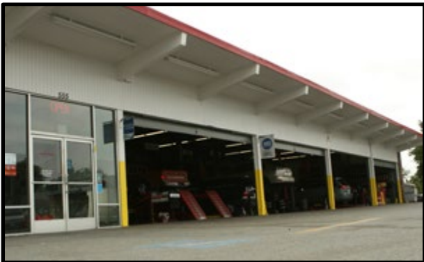
Auto Service Garage
