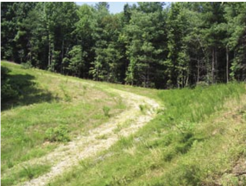
Stabilized forest access road. Note side/cut banks angled appropriately to minimize erosion.
