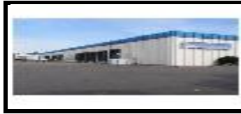
Cold Storage Warehouse
