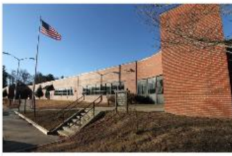
ADMINISTRATIVE SERVICES BUILDING Switchgear Replacement
