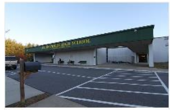
A.C. REYNOLDS HIGH Roofing Projects
